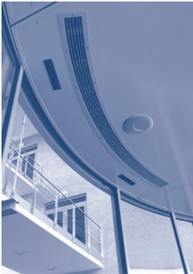
Installed within a suspended ceiling with curved air outlet (non-standard model)
